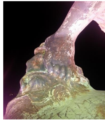
Fig. 11. The corrosion of the statue of victory (2013).
