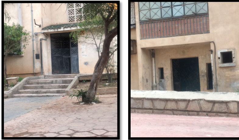
Photos 1/2: The entrance doors of the LSP building Source: Author 2023
